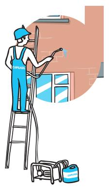
The BEAL technical team recommends in most cases a 2-layered "fresh on fresh" application for optimal product penetration. The next coat pushes the previous one more deeply into the support. It is this depth of penetration that ensures the longevity of the treatment.
